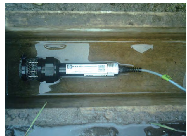
Inside of U-shaped irrigation channel after the cleaning and maintainance
