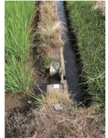
Souma : Water-Intake Gate
