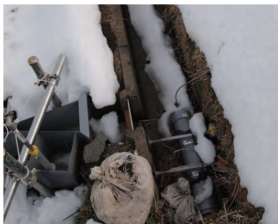
Souma : Water-intake gate
