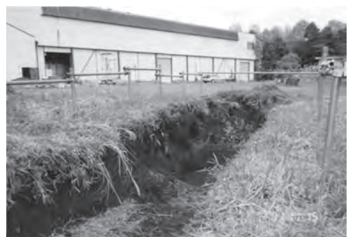
Photo 1 Condition at the trench
